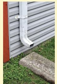
Attach a downspout extender and direct it to the lawn and away from the foundations.
