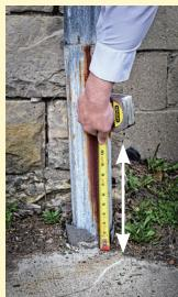
Measure and cut the downspout 10 inches above the ground with a saw.
